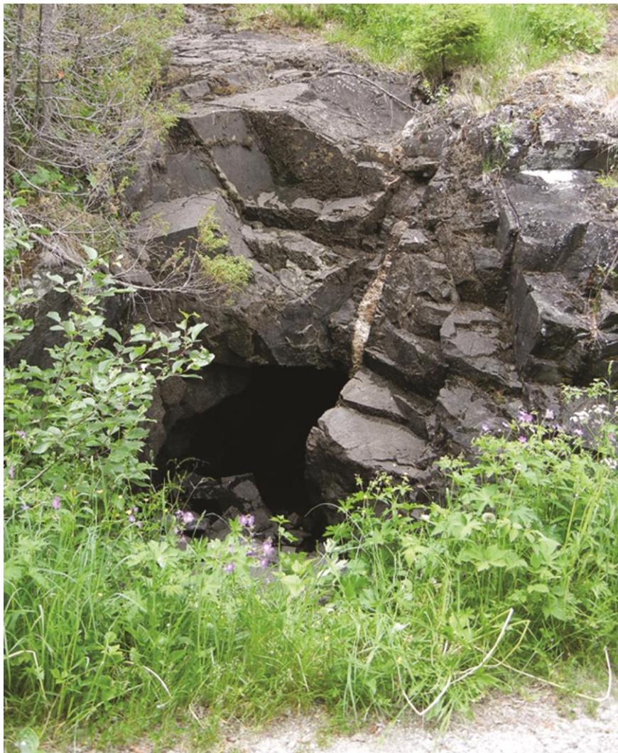
Fig. 1. The entrance of the E-adit at Bleka. The steeply dipping eclarite bearing quartz vein is visible on the right hand side of the adit. Photo: A.O. Larsen.
