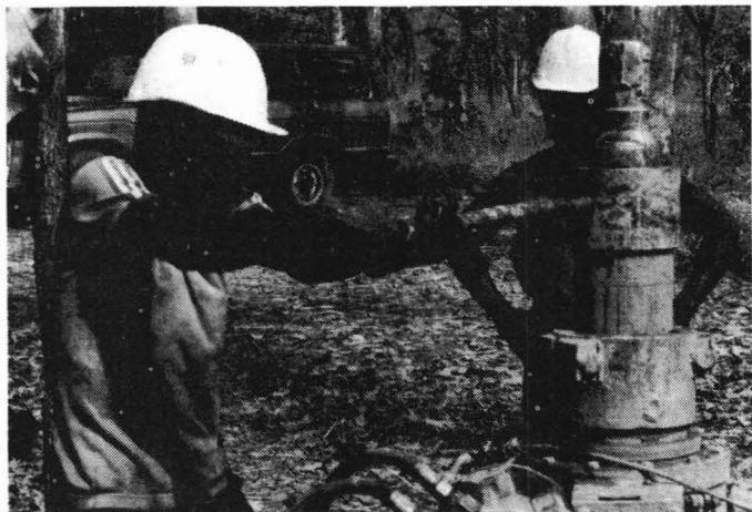
Banka drilling in placer - Banka boring i «placer».
